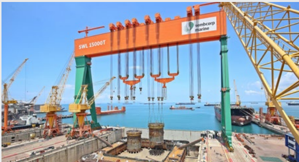
Sembcorp Marine's goliath gantry crane at Tuas Boulevard Yard lifting Shell Vito FPU columns
