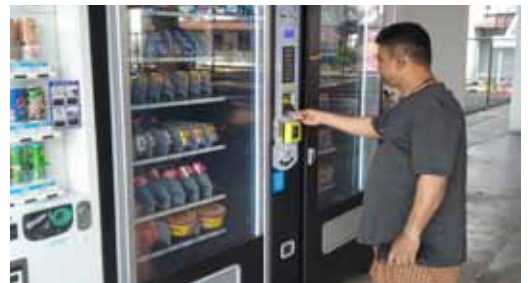
We installed new vending machines and portable water dispensers at our Alaulia Lodge for our migrant workers to grab a snack or drink conveniently
