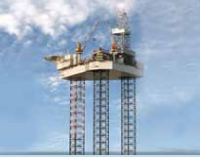
Deep Driller I , first proprietary Pacific Class 375 design jack-up rig
