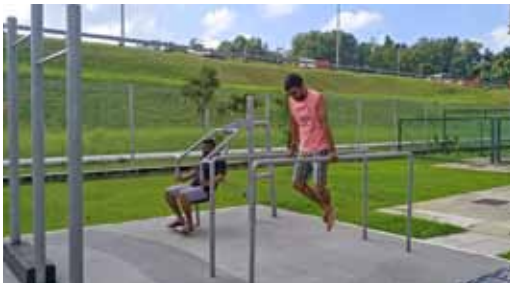
We constructed a new exercise area to promote healthy living
